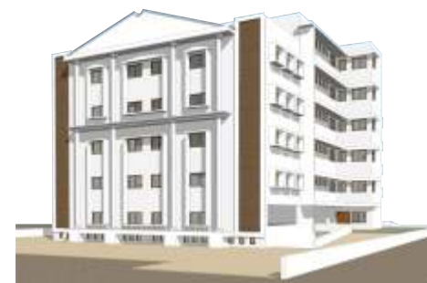
Mihan SEZ, Nagpur (under construction)
